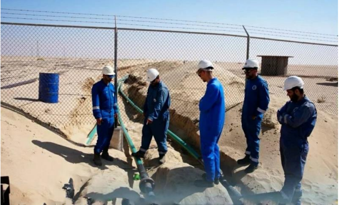
Section of the 1,600-metre composite pipeline connecting well VV-28 to Al-Blat station
